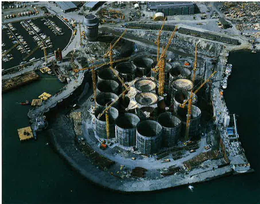
Gullfaks C in dry dock, April 1986 - 4 months after start of construction!
